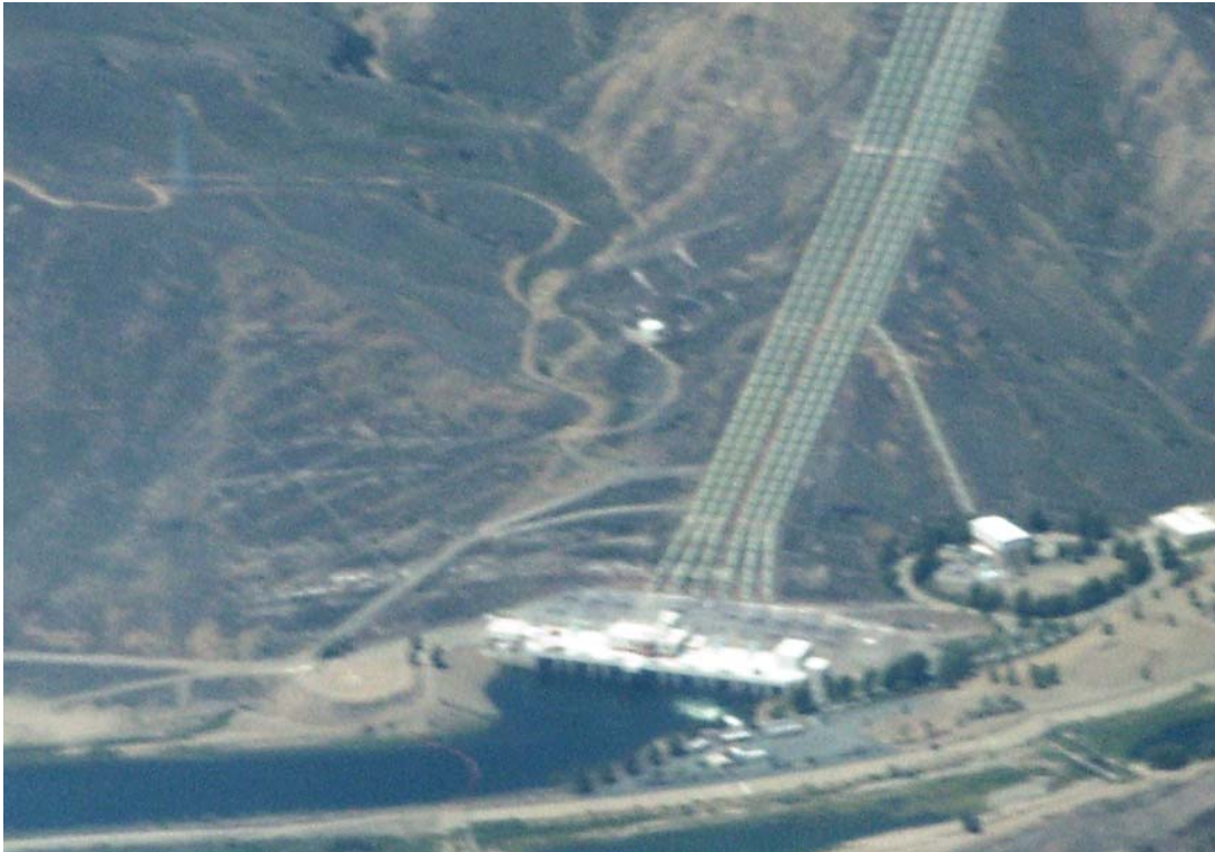
Large water pumping operation in the mountains
